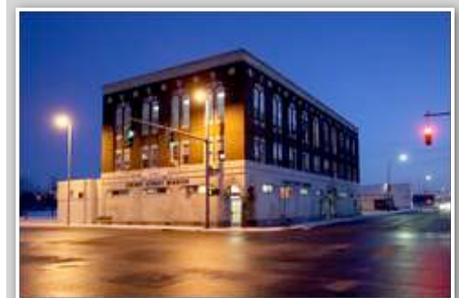
The Cherry Street Mission as dawn approaches and the men inside start to wake up.
